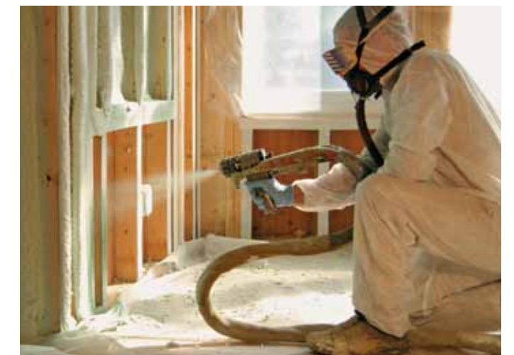
Proper prep yields the best installation. While spray foam is installed by a pro, it's your responsibility to prep the site. Masking windows, electrical boxes, and even floors is important if you want the foam contained to wall, roof, and floor cavities. Anyone on site during the installation should be outfitted for optimum protection.
