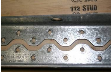
Photo 26: Simpson HDU8 Hold Down
