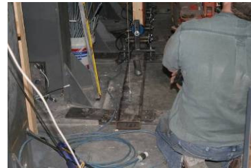
Photo 34: Alignment of Frame
