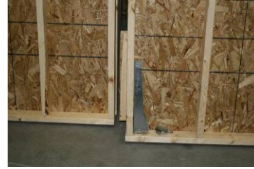
Photo 27: Simpson HDU8 Hold Down
