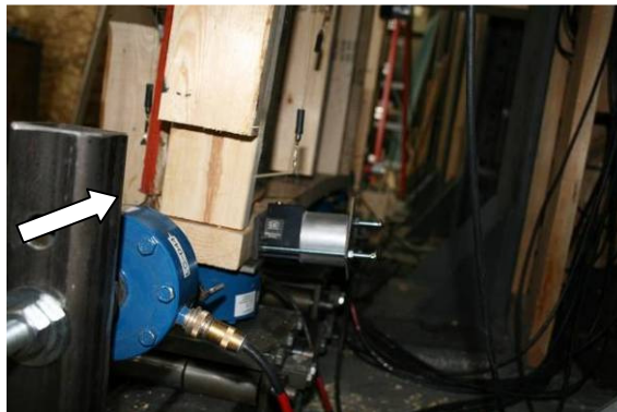
Photo 1: Stud/Plate Separation at Hold Down
