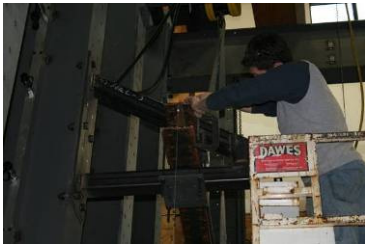
Photo 33: Alignment of Frame
