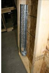
Photo 30: Simpson HDU14 Hold Down
