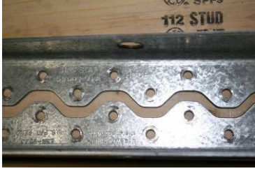
Photo 26: Simpson HDU8 Hold Down
