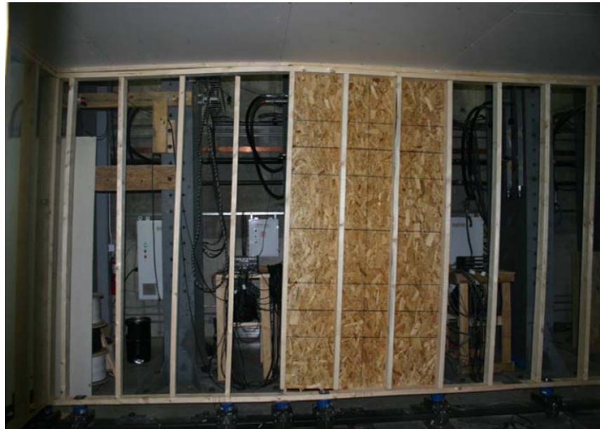
Figure 10: SBCA Research Institute Wall Failure (SBCARI T-IRC)
