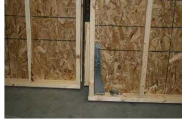
Photo 27: Simpson HDU8 Hold Down
