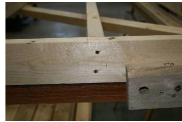
Photo 13: Wall Stud Connection
