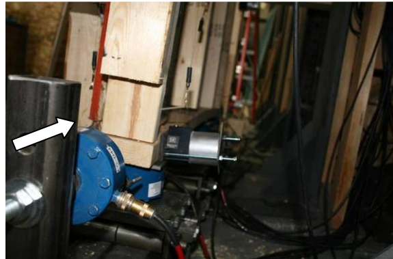
Photo 1: Stud/Plate Separation at Hold Down
