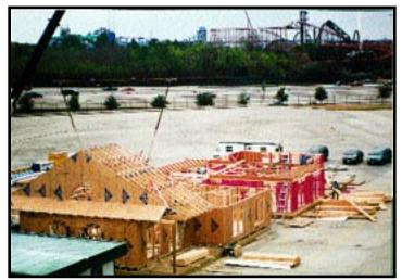
And lead they have! From Framing the American Dream® to the introduction of new and innovative products, the associations and major players have led the way. Framing the American Dream® was the comparison of a component built house to a stick frame built house. The two houses were built side by side during the National Association of Home Builders trade show. This one promotion exposed over 65,000 builders and contractors to
