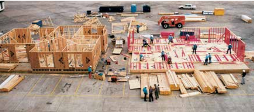
Photo 1. The Framing the American Dream jobsite shows how much more progress (and fewer workers) are by the house being built with structural components (on the left) compared to the house being built with stick framing (on the right).
