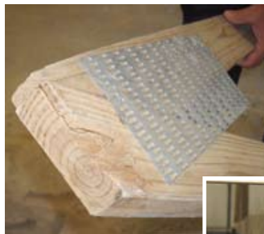
Damage to the actual truss on the jobsite. It shows splitting at the end of the bottom chord.
