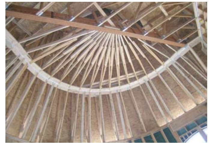
The tower is framed with high-heeled scissor trusses, creating a true conical roof shape. Scabs added to the sides of many truss bottom chords create an alternating straight and curved shape at the top of the wall. This makes way for the transition to a true continuous circle for the tower. A total of 15 trusses with a 28/12 pitch create a “fan effect,” said Kolosky. The trusses tie into the angled beam (top).
