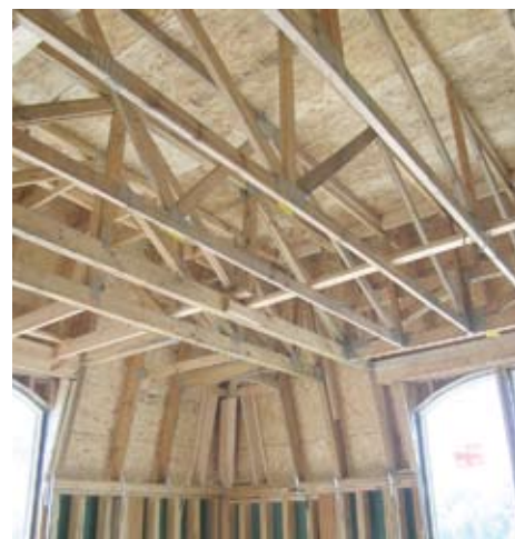
View of loft corner. The top left shows jack trusses tying into the main east-west trusses to provide stability to the walls. (The framing and straps tying the jack trusses to the main span trusses are not yet in place.)
