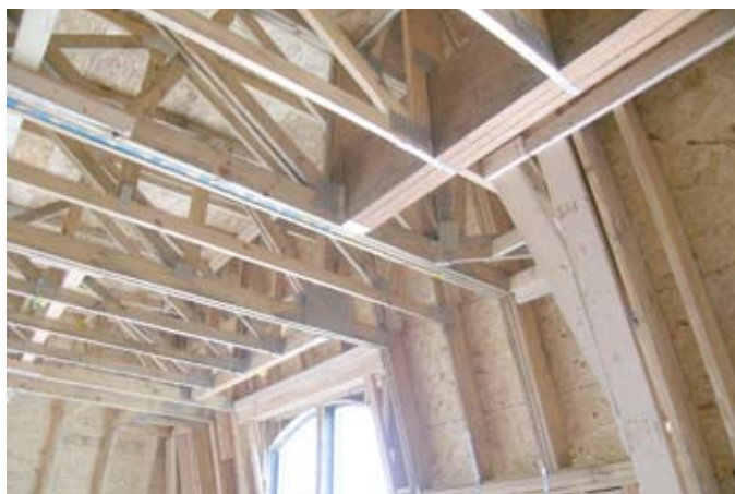
The short span roof beam hanging on a girder tray truss. Also, a header truss at the dormer supported by a tray girder truss at each side of the dormer.
