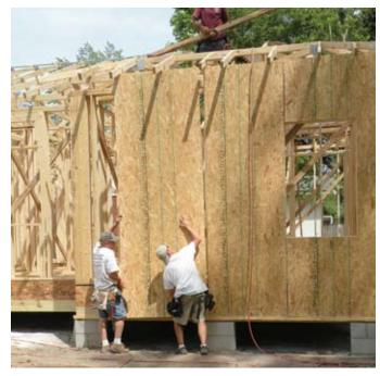
Wall Sheathing. Instead of horizontal wall sheathing, 11' vertical sheathing panels run continuously from the top plate to the bottom plate. This technique minimizes energy loss that occurs in the horizontal seams. "The longer panel lengths allow a single sheet to be installed from the roof trusses to the support beam in the floor system. It removed the cost of the typical wall uplift connectors and various blocking requirements," Kozlowski said.
