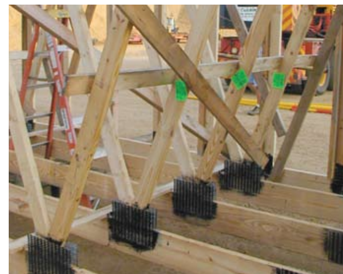
Install Web Member Permanent Lateral Restraint and Diagonal Bracing (or web reinforcement) and Bottom Chord Permanent Lateral Restraint and Diagonal Bracing as required.
