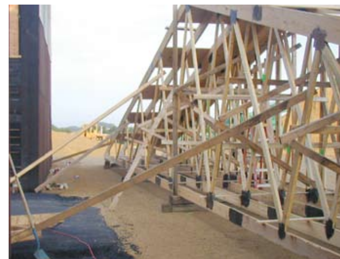
Ground Bracing for truss assembly being built on the ground.
