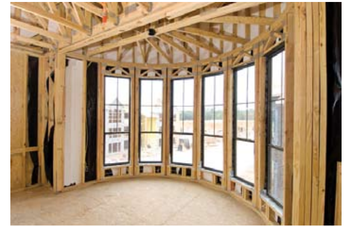
Harris says like traditional wall, roof and floor components, its plated headers, corners and other rough openings offer builders and framers tremendous value in many areas.
