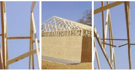
While traveling through southern Georgia, Glenn Traylor (ITW Building Components Group) ran across this project. The entire building is braced with ripped 1/2" x 2" x 24" OSB. "If the typical 2 x 4 or 1 x 4 braces are 'killer cleats' then this needs a new description." he said.
