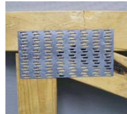
Figure 2. Pitch-pocket under plate area.
