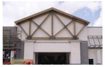
a truss that big in our facility, disassembling it completely [for shipment], and then reassembling it on the jobsite, without problems." After the trusses were built in the shop, they were pressure treated and then shipped to the jobsite in pieces, said Lincoln.
