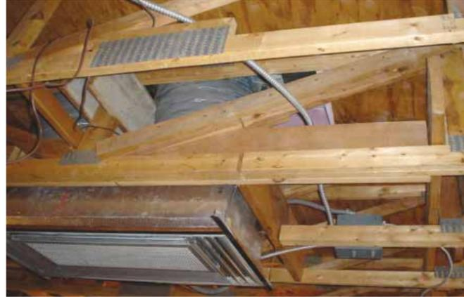
lbs. sitting directly on the trusses. Despite the incorrect alterations and the snow, ice and rain loads for the last 15 years, the trusses held up without any noticeable problems. The CM, who asked not to be named, was very surprised that the structure lasted this long, especially given it was a clear-span flat roof with no interior walls.
