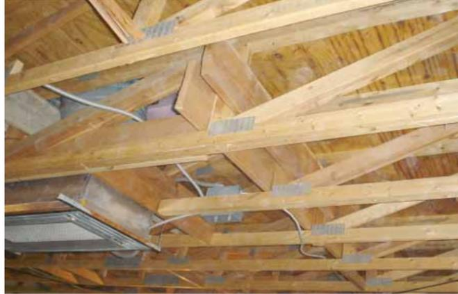
One WTCA member sent in these pictures of cut girder trusses discovered during the remodel of a local restaurant. A contractor who works regularly with this component manufacturer was doing interior remodeling and re-roofing on the restaurant when they noticed a previous contractor had cut some of the girders. The contractor recognized the problem and immediately contacted the component manufacturer.
