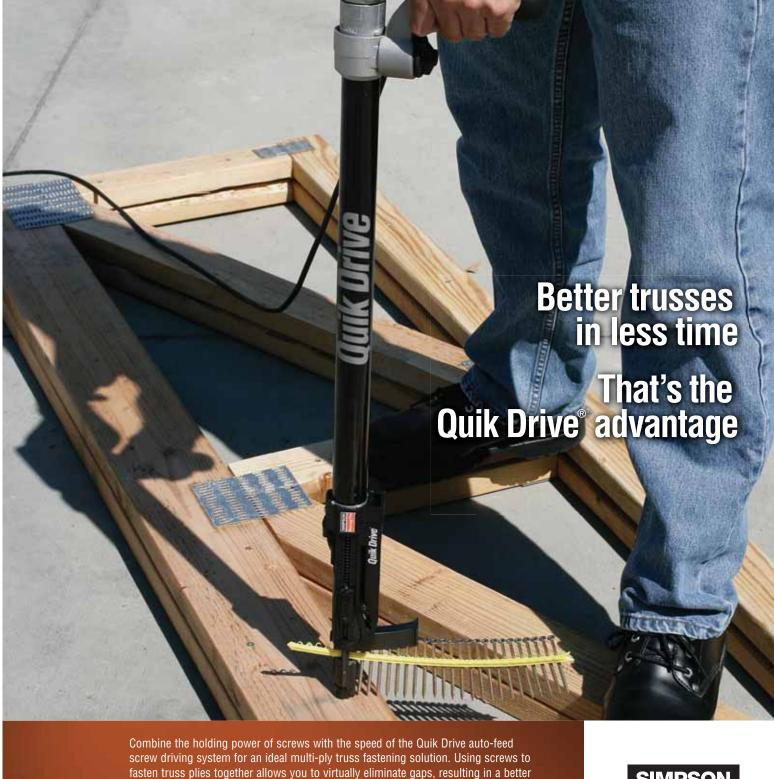
finished product. And since the Quik Drive system features collated screws and our patented auto-feed mechanism, your crews can continue to work as fast as ever while potentially reducing injuries when compared to nail gun users. Now doing the job better doesn't have to take more time.
