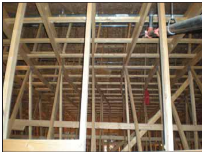
Photo 1. Buckled top chords of supporting trusses in piggyback system resulting from a failure to install diagonal bracing in top chord plane.
