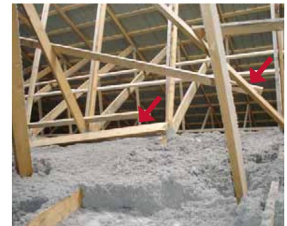
Photo 1. Example of broken compression webs in which the CLR was attached but had no diagonal bracing. The red arrows point to the broken webs in two adjacent trusses. Note that the CLR is still attached to one of the webs.
