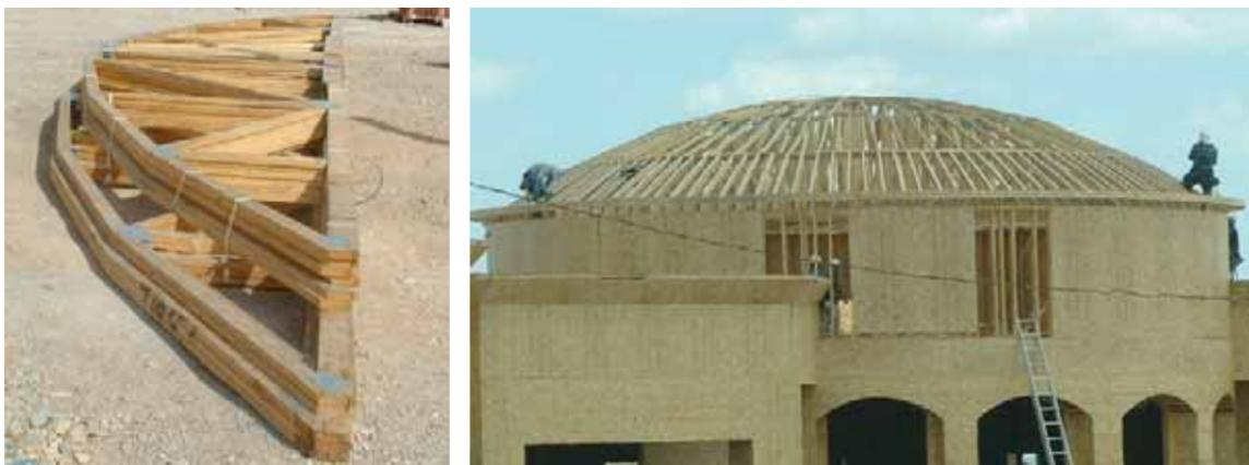
This recently completed retail building in Las Vegas, NV features bow-string trusses. Justin Henricksen, a truss technician in the Las Vegas area, designed the trusses for the domed structure. Henricksen says he has been seeing quite a few requests for the bow-string trusses, although this one was their biggest so far at 58'. He commented, "Everybody wants to do these round towers, it seems to be the norm right now."
