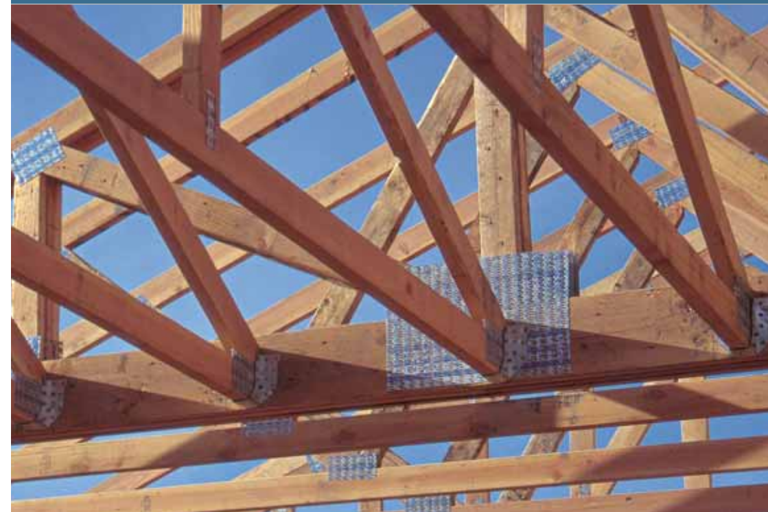
THGQ/THGQH High Capacity Girder Truss Hangers
