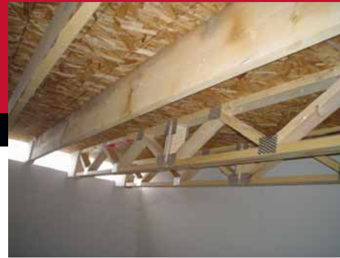
The floor assembly had 2x10 SPF joists and 12" floor trusses spanning from the low end to the high end. These were sheathed with 23/32" OSB. Joists and trusses were included in the same structure so they would be exposed to identical fire conditions.
