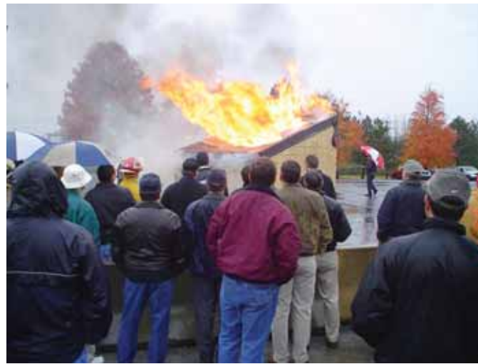
At 13 minutes, 19 seconds, the trusses and joists collapsed simultaneously. This demonstrated that trusses and joists, when equivalently loaded, perform similarly in fire. It also showed that unprotected construction will not last long in fire.
