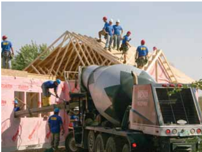
Coordination is key for any Extreme build. At the Richco site, sheathing was applied to the garage roof while concrete was poured for the basement below.
