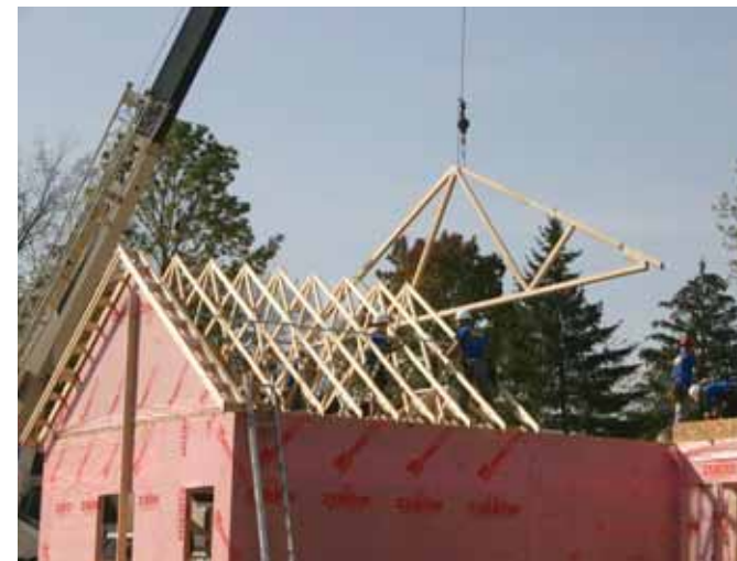
Roof trusses for the garage being set on the Richco site.
