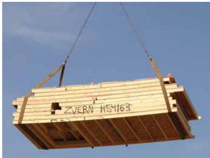
Wall panels were hoisted to the second floor of the building on the Richco site.
