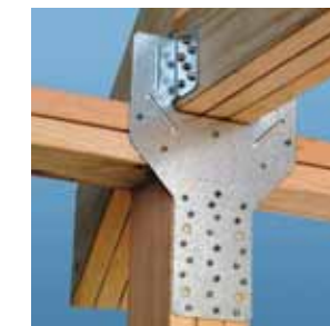
LGT3 3-Ply Girder Truss Tiedown
