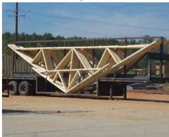
Roof trusses are stacked vertically on a custom-built trailer.
