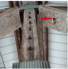
Figure 3. Sections of OSB sheathing between the members of the trusses on each side of a pole have been used as bracing for the bottom chords and webs.
