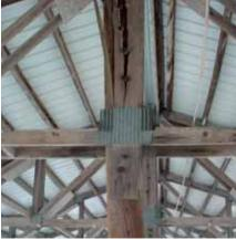
Figure 2. The trusses are a double Pratt design with 2x6 top chords and 2x4 bottom chords constructed of Southern Pine. The chords are all #1 grade and the truss plates 20 gauge. The distance from the concrete slab to the bottom of the trusses measures 15.5'. The 2x8 kingposts extend 14" through and below the bottom chord to allow for more bolts. Each pair of trusses is bolted to their pole with eight 3⁄4" diameter bolts more or less evenly spaced down the kingpost.
