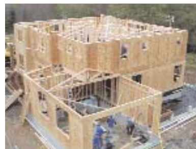
1 st Floor Wall Panels, 11 am-12 pm: Exterior Deck Frame, 11 am-12 pm: 2 nd Floor Panels/Stairs, 12-1:30 pm: 2 nd Floor Wall Panels, 1:30-4:30 pm: Covered Porch/Columns, 1:30-6 pm: Roof
