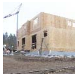
1 st Floor Wall Panels, 11 am-12 pm: Exterior Deck Frame, 11 am-12 pm: 2 nd Floor Panels/Stairs, 12-1:30 pm: 2 nd Floor Wall Panels, 1:30-4:30 pm: Covered Porch/Columns, 1:30-6 pm: Roof
