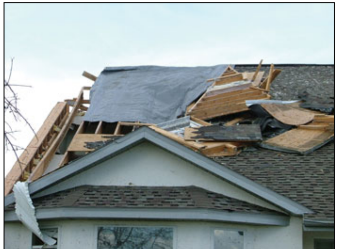
This house shows that both roof trusses and I-joists are susceptible to damage in a hurricane.
