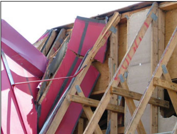
At an Arby's restaurant in Port Charlotte, the sign fell off and hit the roof, breaking one truss member. These façade trusses performed well during the storm due to connections and bracing.
