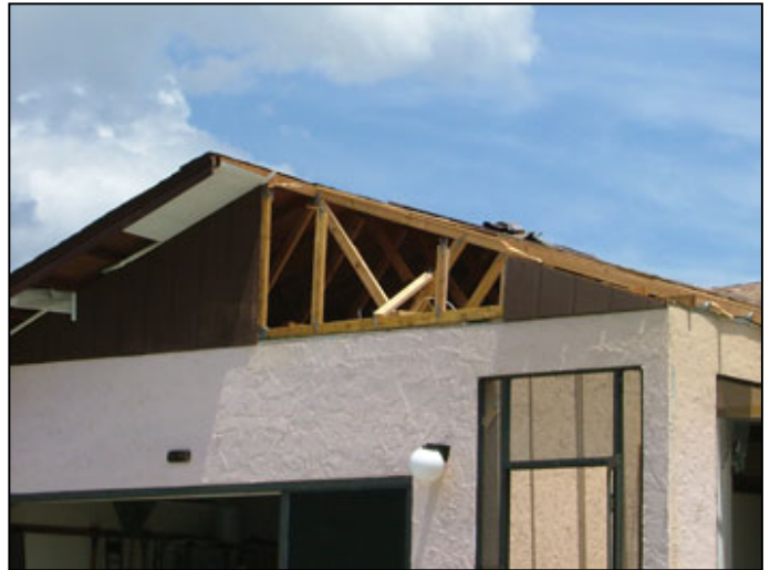
This home was built in 1979 and suffered substantial roof damage as wind blew out all the gables and the roll-up shutters on the lanai. However, the connectors between the trusses and walls performed quite well.
