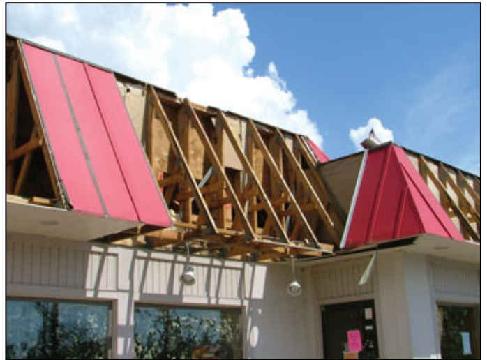
At an Arby's restaurant in Port Charlotte, the structure's truss damage was minimal. Notice that the façade bracing was good.
