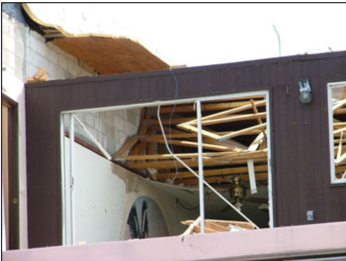
This condominium was built between 1960 and 1970. There is no evidence that the trusses were anchored to anything, and no connections or bracing.
