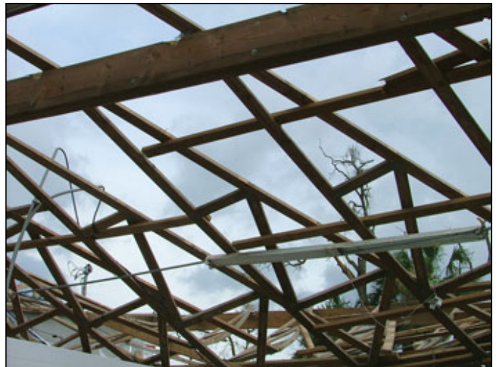
Post frame building with no sheathing; purlins blew off and connected properly and no permanent bracing.
