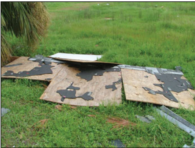
Sheathing ripped off roof.
