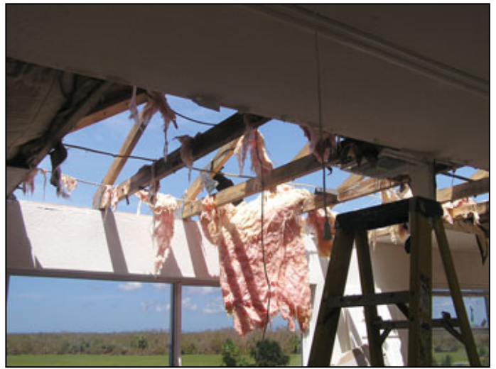
This home was near completion in the Pine Island/Port Charlotte area and the homeowners were days away from moving in. The roof trusses held their ground.
