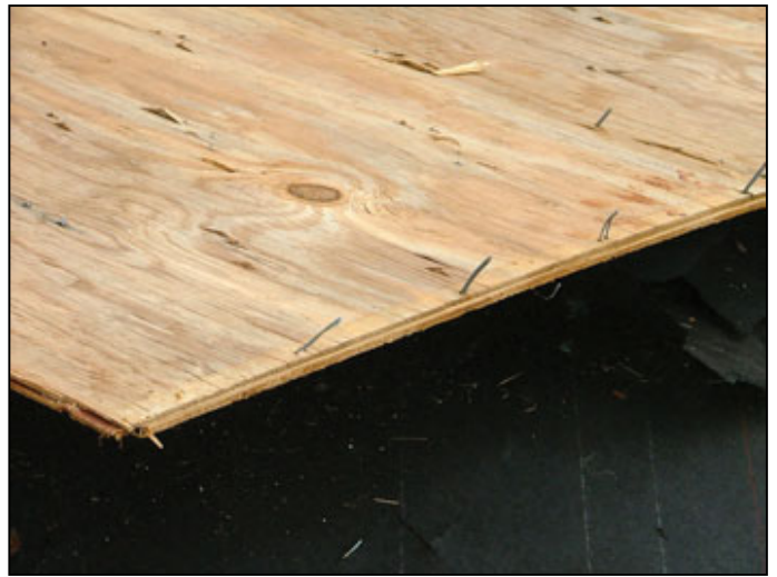
Sheathing fastened with nails and staples.
