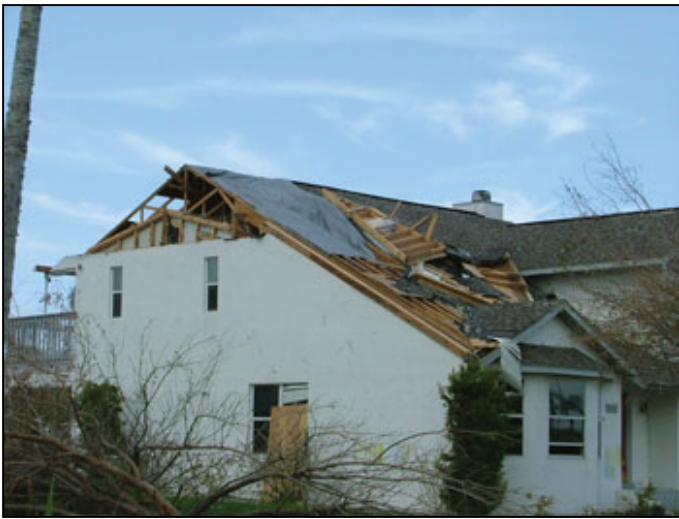
This home built in 1984 sustained considerable roof damage. Again, the truss connections to the wall framing performed well.
