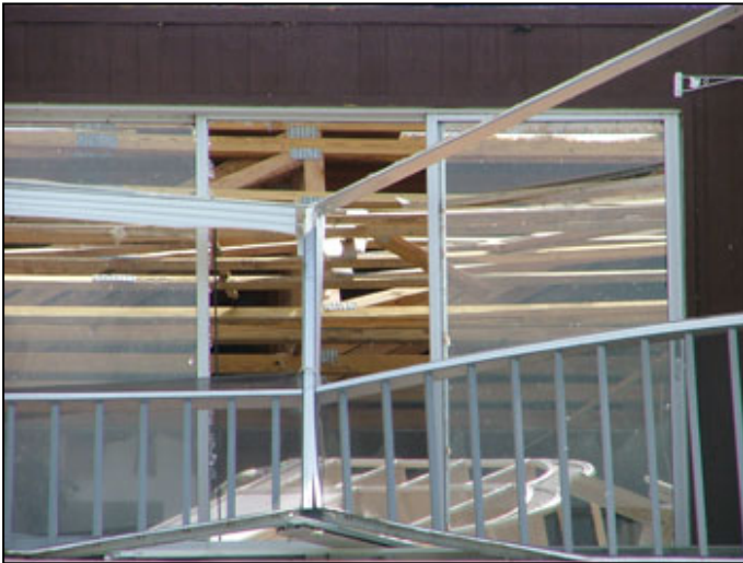
This condo was built in the 60s or 70s, next to Charlotte Harbor. There was no evidence of permanent web member bracing in the roof system and obviously, the plywood roof sheathing was not nailed in place to resist the uplift forces.
