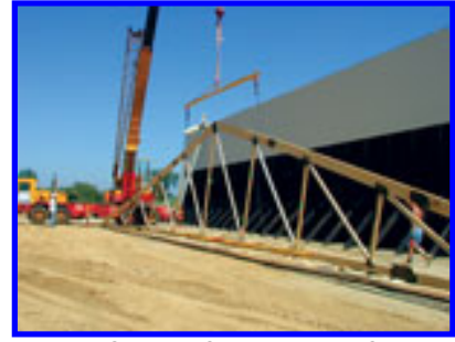
LIFTING DEVICE MADE PICK-UP FAST, SAFE AND EASY.
