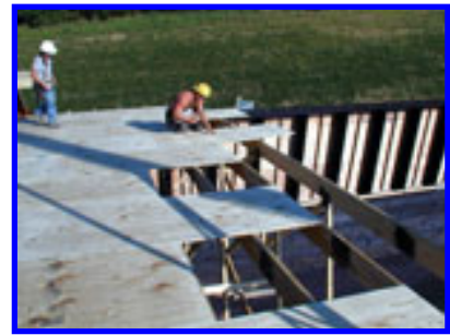
PERMANENT BRACING—SHEATHING AS TRUSSES WERE INSTALLED MADE ENTIRE SYSTEM RIGID.
