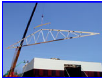
LIFTING DEVICE KEPT TRUSS RIGID IN AIR AND THROUGHOUT INSTALLATION.
