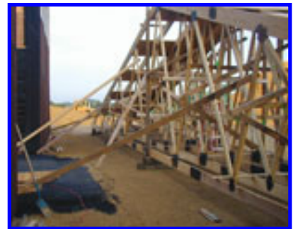
GROUND BRACING ON FIRST FIVE AFTER BEARING TIMBERS ARE LEVELED.
