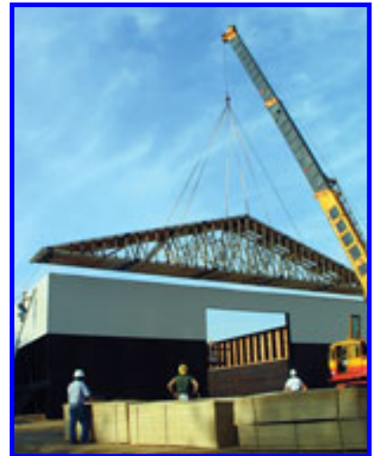
HOISTING FIRST FIVE SYSTEM, LINING UP TO EXTERIOR WALLS.
