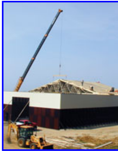
EACH TRUSS TOOK ABOUT 15-20 MINUTES TO INSTALL AND BRACE.
