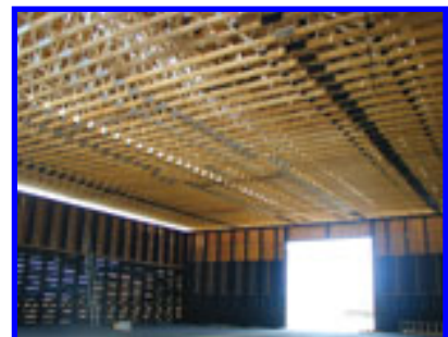
INSIDE OF COMPLETED SALT STORAGE FACILITY.
