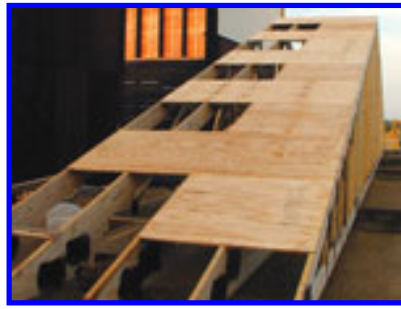
SHEATHING ON FIRST FIVE, ALTERNATING 4X4 AND 4X8 SHEETS.
