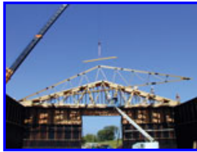
NEW LIFTING DEVICE EASED INSTALLATION.
