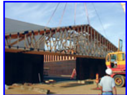
LIFTING FIRST FIVE SYSTEM—NOTE THE THREE PICK POINTS.
