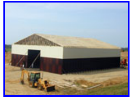
INSTALLATION COMPLETE; TOP CHORD SHEATHED.
