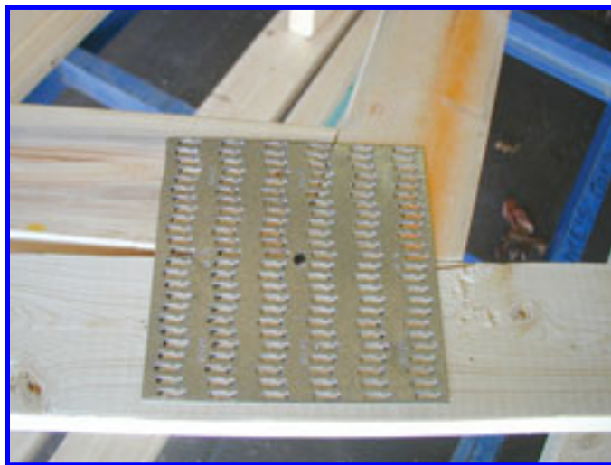
FIGURE 3. UNDER TCM, PLATE POSITIONING IS JUST ONE OF FOUR NECESSARY CHECKS.
