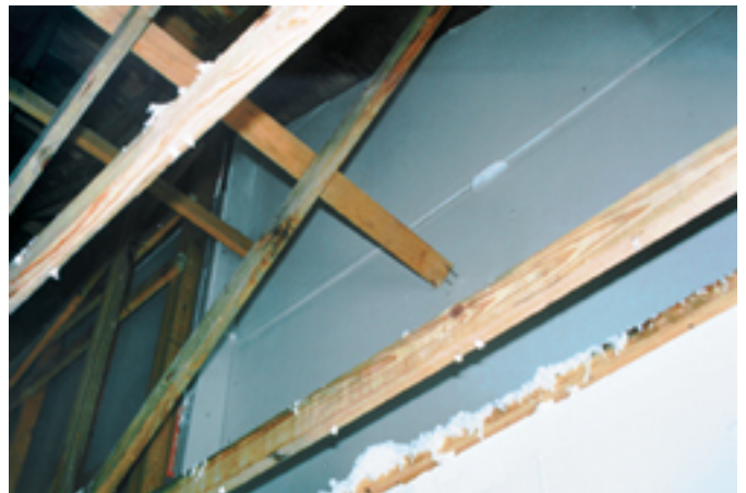
Figure 3. These 4x2 floor trusses were not fastened properly. The vertical anchor from the tie beam was misplaced, and only a few nails hit the wood. The strap was misplaced by three inches and was bent down onto the tie beam and up at the truss.
