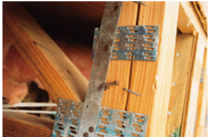
Figure 3. These 4x2 floor trusses were not fastened properly. The vertical anchor from the tie beam was misplaced, and only a few nails hit the wood. The strap was misplaced by three inches and was bent down onto the tie beam and up at the truss.
