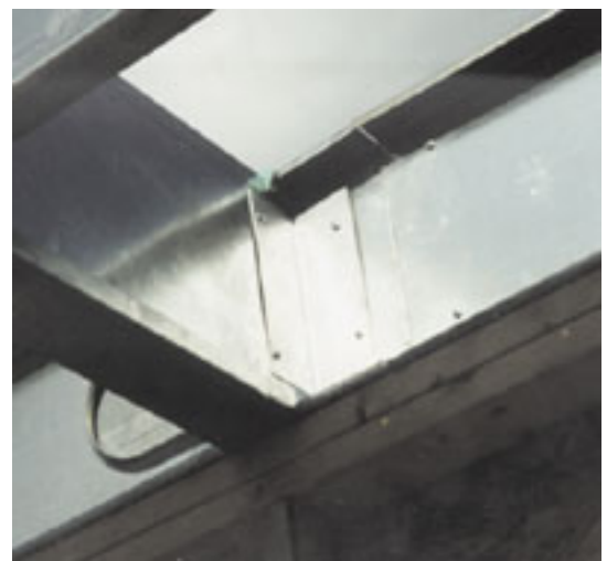
STEEL FLOOR JOISTS REST ON TOP OF WOOD FRAMED WALLS
