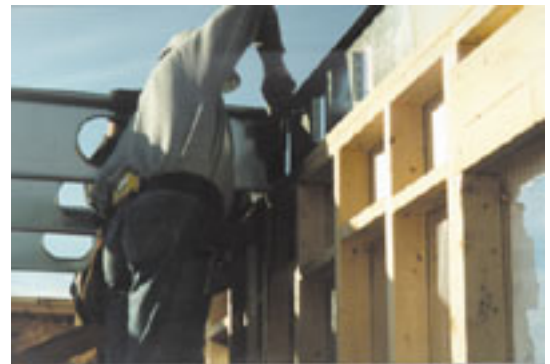
A WORKER ATTACHES STEEL FLOOR JOISTS
