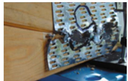
Shear failure at a heel joint on one of the tested trusses after loading.
