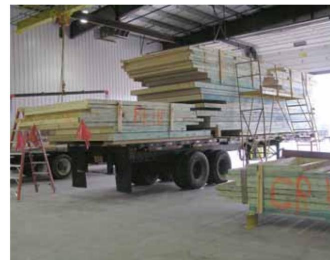
Walls are loaded on the delivery truck so framers can work in sequence, eliminating the need for double handling.
