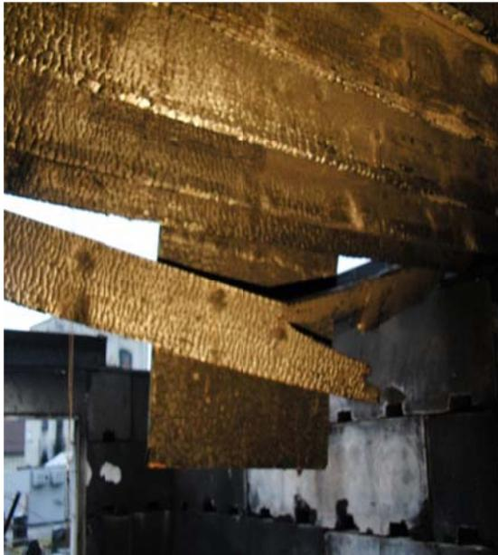
**Figure 46. Dimensional Lumber Joist Fracture**
