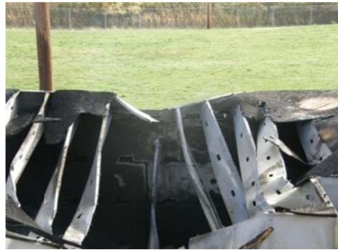
**Figure 53. Steel C-joist deformation detail**
