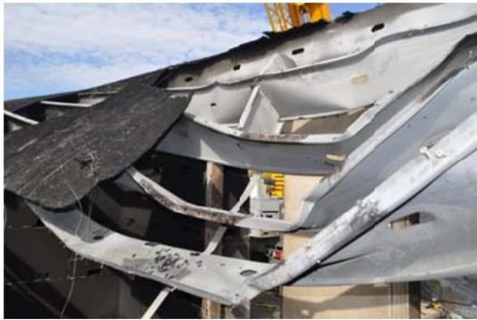
**Figure 52. Steel C-joist Loss of strength inducing progressive joist deformations, sheathing connection failure, joist bracing and lateral bracing strap failure**
