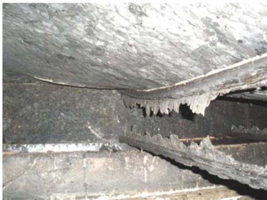
**Figure 48. Engineered I-joist Web Burn Through**
