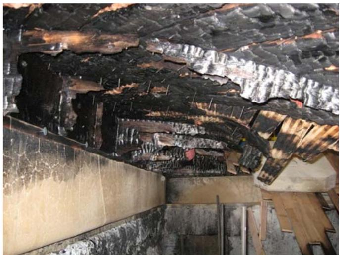
**Figure 47. Dimensional Lumber Complete Joist Burn Through**
