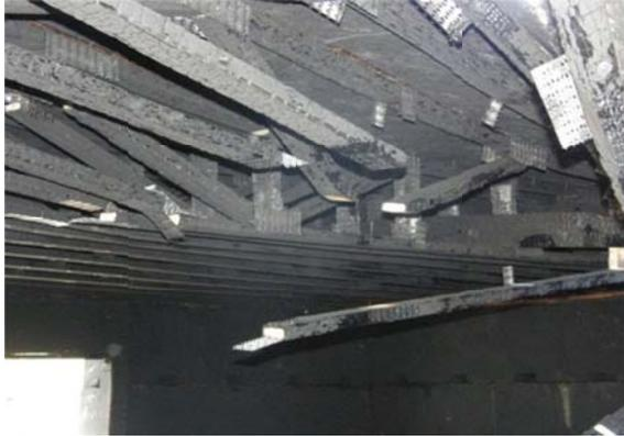
**Figure 50. MPCWT Steel to wood panel point connection failure**
