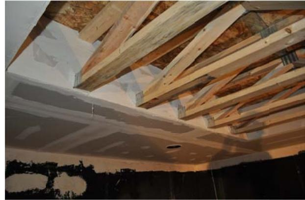
Figure 57. Detailed image showing draft stopping of the exposed trusses
