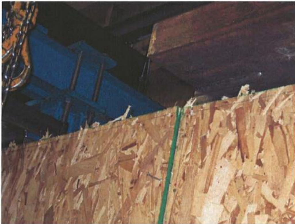
Figure 8: Typical OSB sheathing edge tearout
