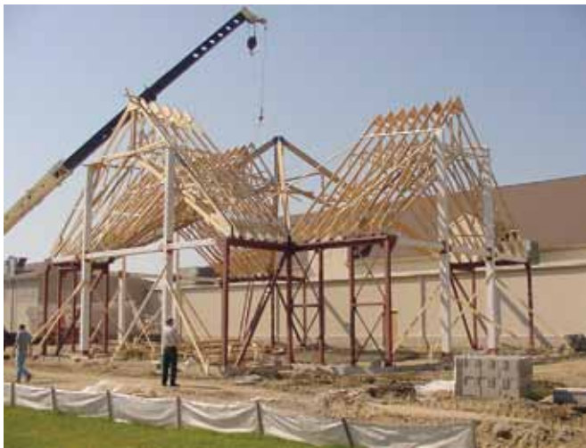
Photo 1. Example of field-spliced scissors trusses.
