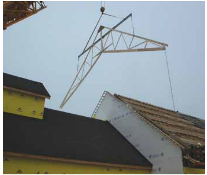
Photo 2. Example of a field-spliced scissors truss being lifted into place.
