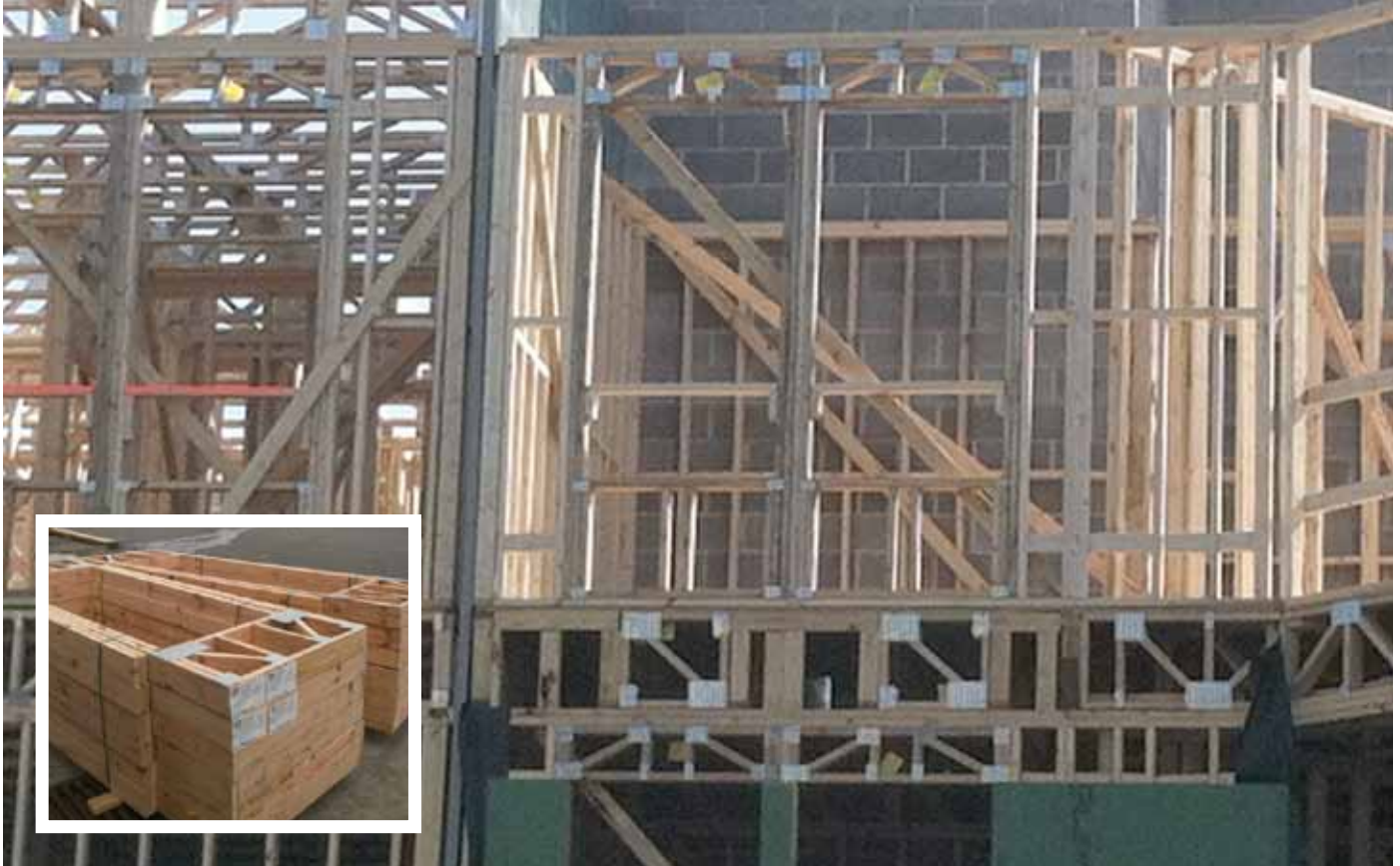
Above: Trussway Rough Openings (TROs) installed on the jobsite help contractors achieve additional green building points. Inset: TROs coming off the production line at Trussway.
