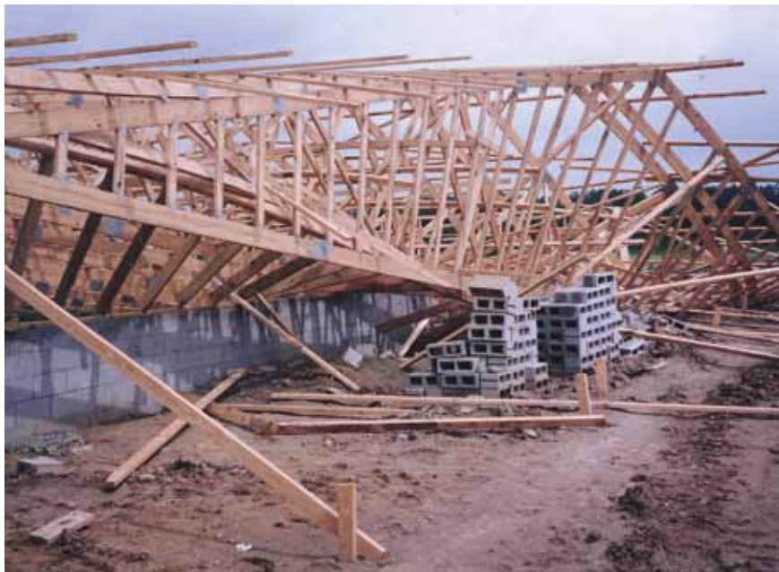
The best time to develop a plan for dealing with a truss collapse is before an accident.
