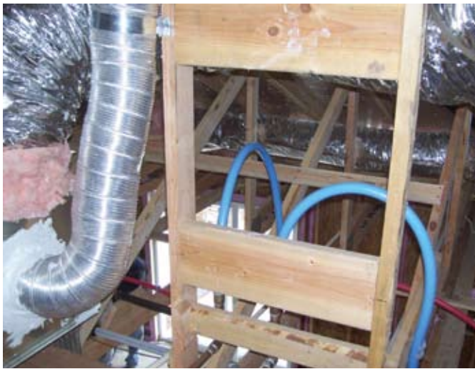
A tankless water heater is mounted to truss verticals. Utilizing this extra space in the attic meant the hot water lines could be limited to 20 feet or less.
