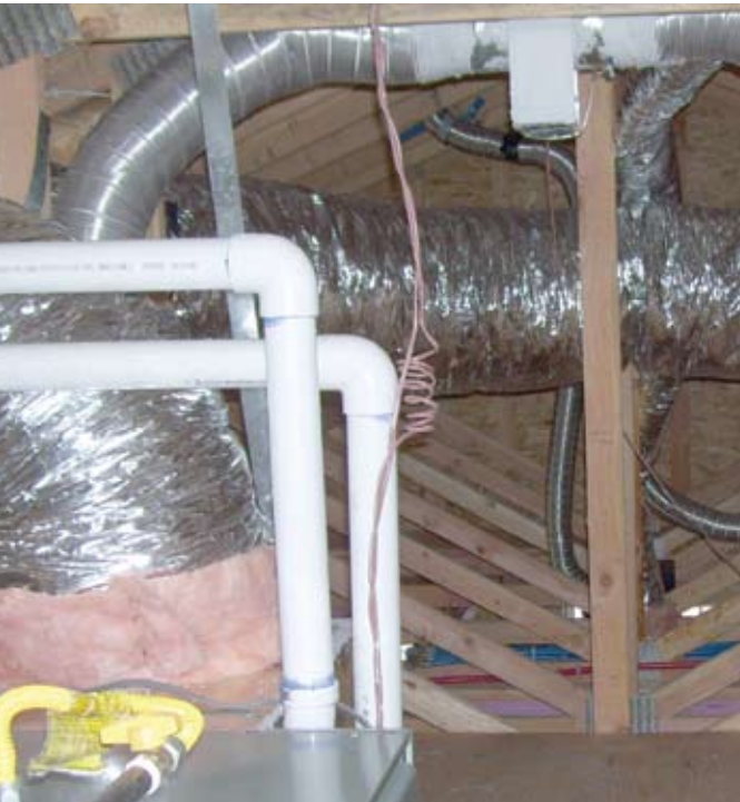
Raised heel trusses provide additional space for fresh air ducting. Outside air passes through a filter, circulates through this mechanical system and into the house.
