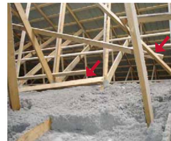
Photo 1. Example of broken compression webs in which the CLR was attached but had no diagonal bracing. The red arrows point to the broken webs in two adjacent trusses. Note that the CLR is still attached to one of the webs.
